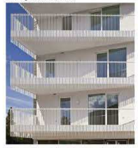
Bermondesey Island, Southwark Metal balustrade to balconies facing park
